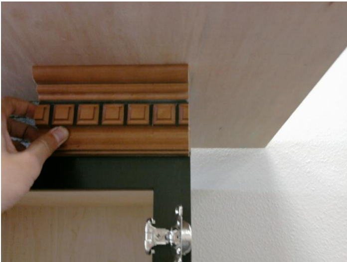
CCM10-B is 3" So make sure to leave 3" for molding.
