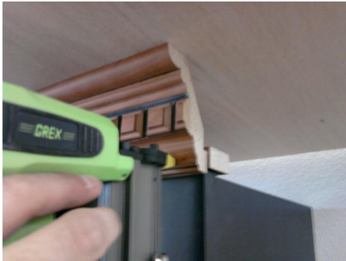
Apply the Molding in front of the wood block
