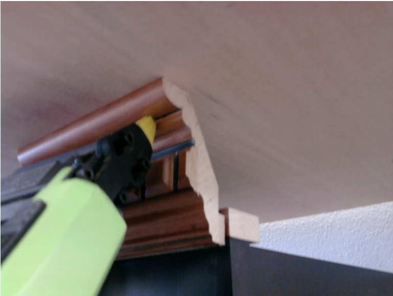
Use 18 or 23 Gauge to nail the molding. Finished!
