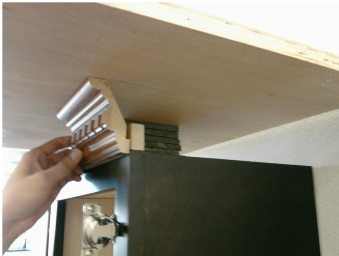
Apply the Molding in front of the wood block
