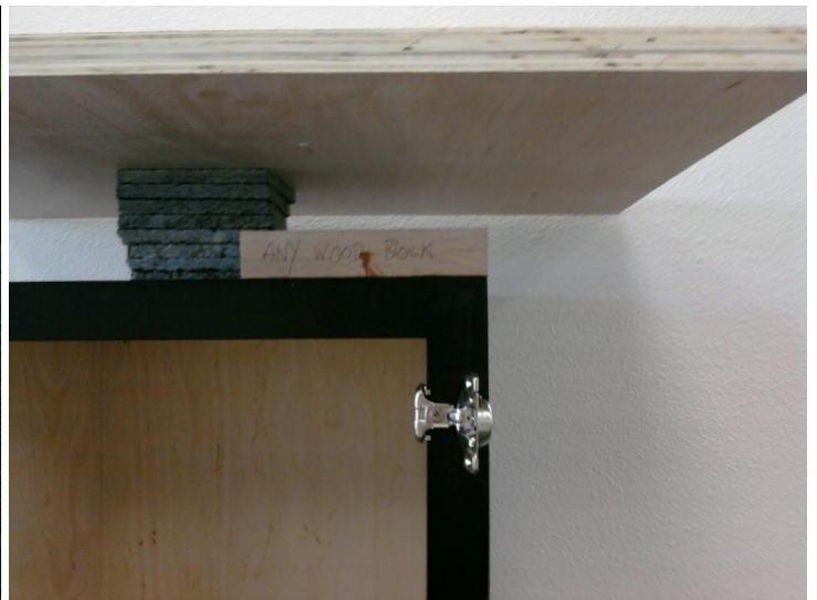
(Cut the back end piece, Leave 1/4-1/2")
